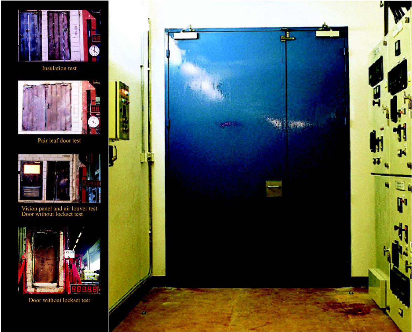
1/2 hr heat insulation and 4 hrs integrity fire rated steel door.
